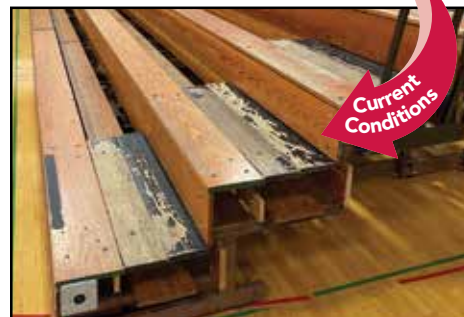
The wooden bleachers at the HS gym are no longer manufactured or utilized, as they pose safety concerns (e.g. no handrails).
